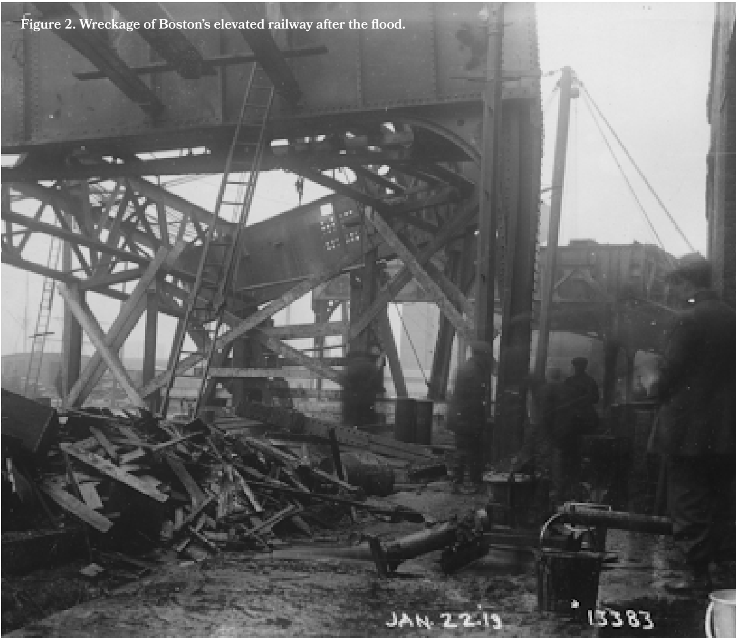
Figure 2. Wreckage of Boston's elevated railway after the flood. This debris was responsible for many of the injuries sustained.
